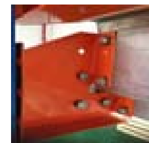
Guide rail junction plate, with good bearing strength.
